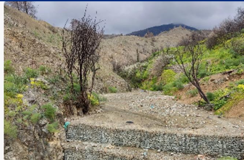
Gabion pond filled-up with materials from the upper watershed
