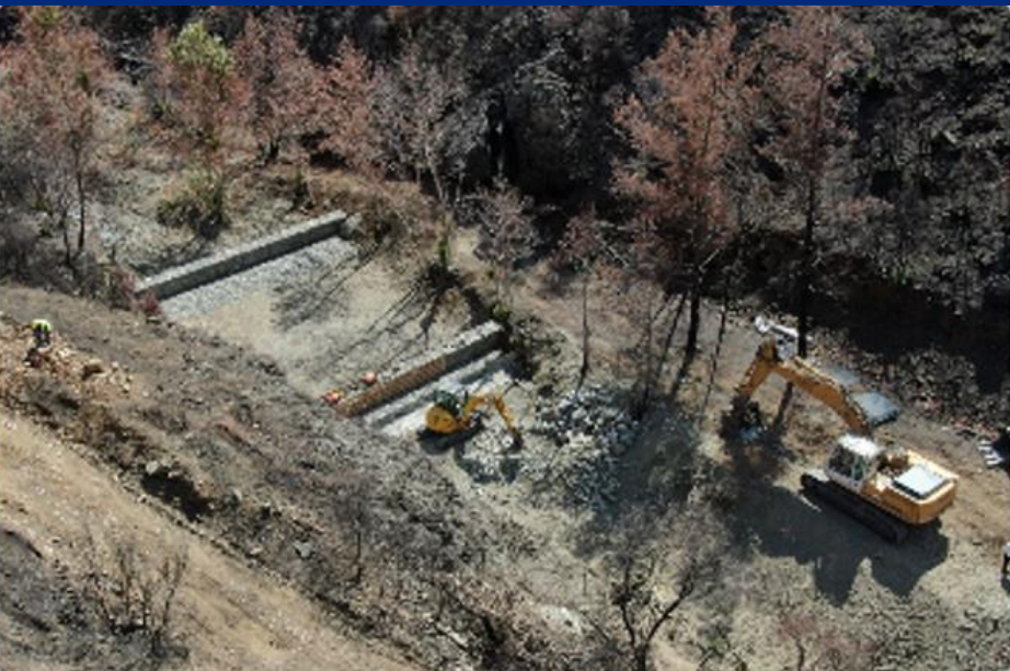
Construction of gabion retention ponds on stream post Arakapas fire, 2021
