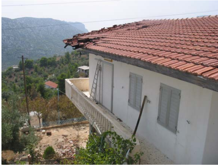
Figure 1. Damaged roof on a house at the base of Parnis mt (Fili) (27/8/2002). The house was saved by firefighters. The owner was not present.
