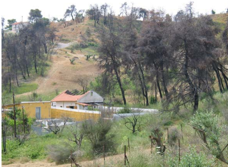
Figure 2. Destroyed home at Bafi, N. Attica (4/6/2001). The roof was the weak point where the fire entered the house.
